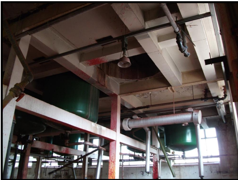
Fig 16: Interior view of (Site 10a) showing the base of the tanks used by European Colour Pigments, looking NW.
