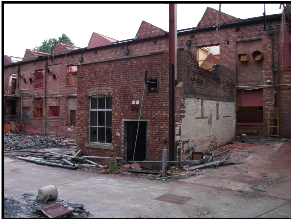
Fig 14: View of the Pumping Station (Site 13) within the Brewery Yard (Site 9). Looking NE.
