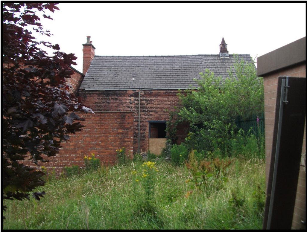
Fig 17: View of late 19 th century Brewery Structure (Site 26), looking N.
