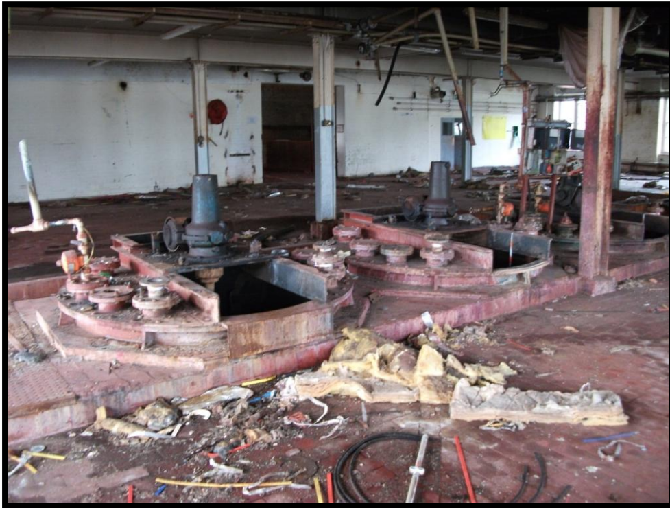
Fig 15: Interior view of (Site 10a) showing the top of the tanks used by European Colour Pigments, looking SW.
