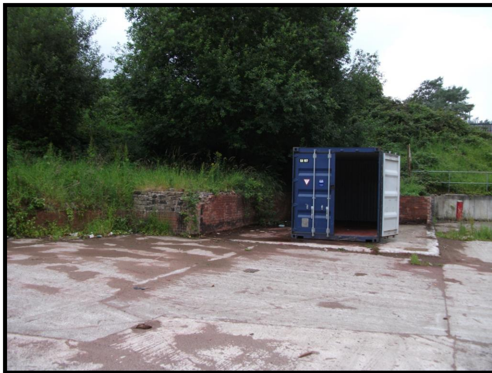
Fig 18: View of Rear Yard (Site 15) and Tank Building Platform (Site 16), looking W.
