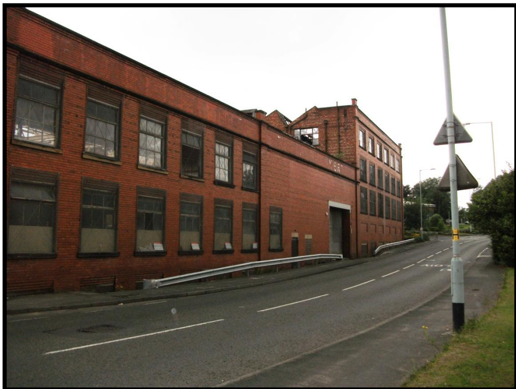
Fig 20: Northern Elevation of (Sites 10a, 10b & 12), looking
