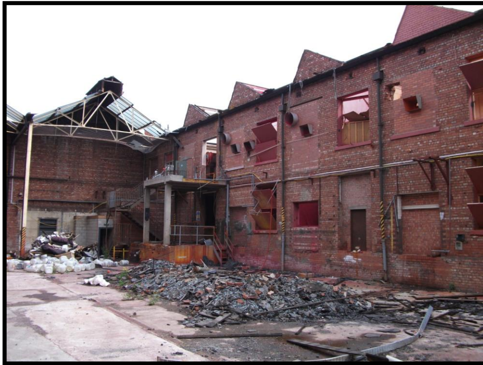
Fig 13: Western Elevation of Bottling Store (Site 12) and Eastern end of Brewery Yard (Site 9), looking NE.
