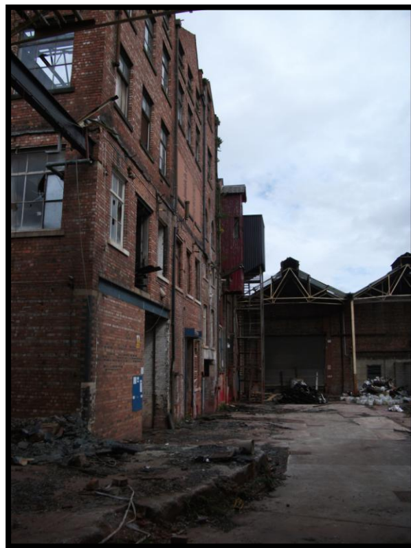
Fig 12: Eastern Elevation of Hempshaw Brook Brewery (Site 10a) and Western end of Brewery Yard (Site 9), looking N.
